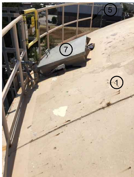
U RAILING AND HATCH
