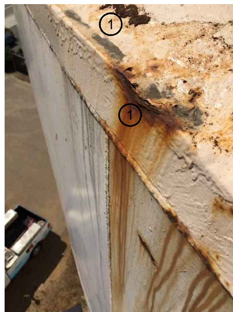
W ROOF PERIMETER
