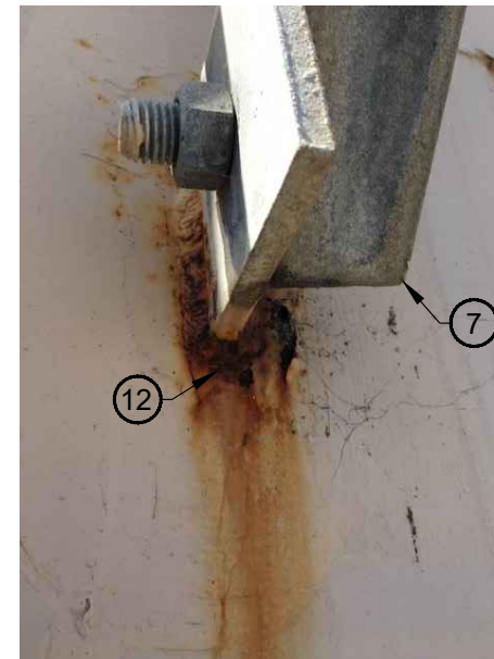
N LADDER SUPPORT CLOSE-UP
