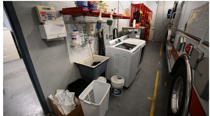
Washer and Dryer in Apparatus Bay
