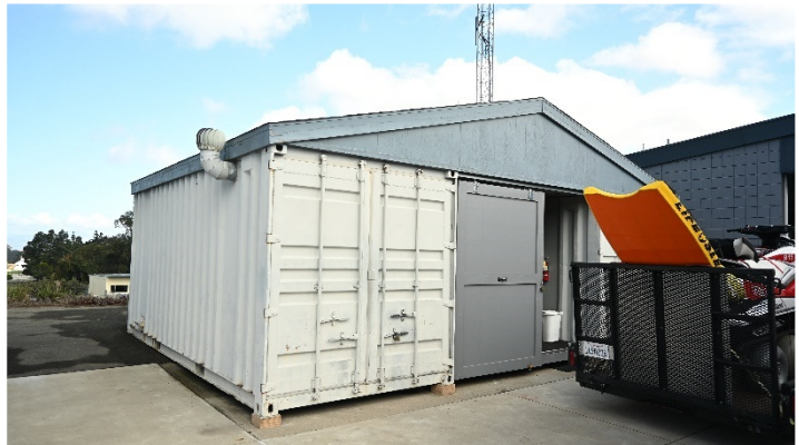
Two C-Trains with Roof Spanning Space for Workshop
