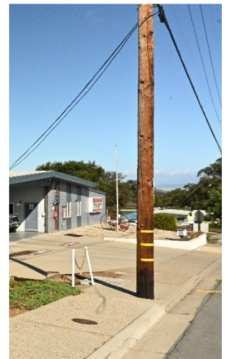
Power Lines Span two Power Poles in Front of the Apparatus Bay
