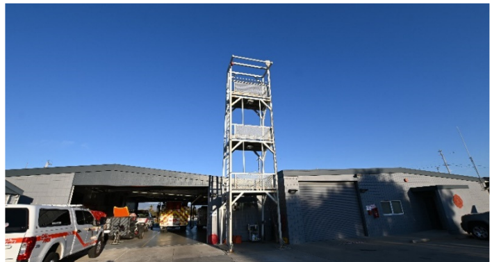
Existing Hose Drying Tower at the back of the Apparatus Bay
