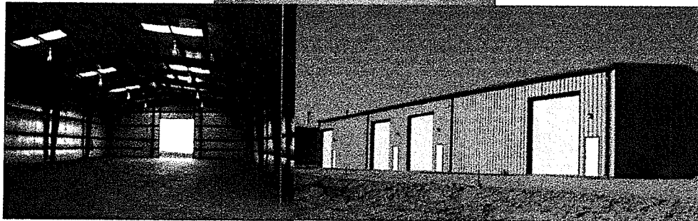
Mojave Wind Park Shop Building Construction
